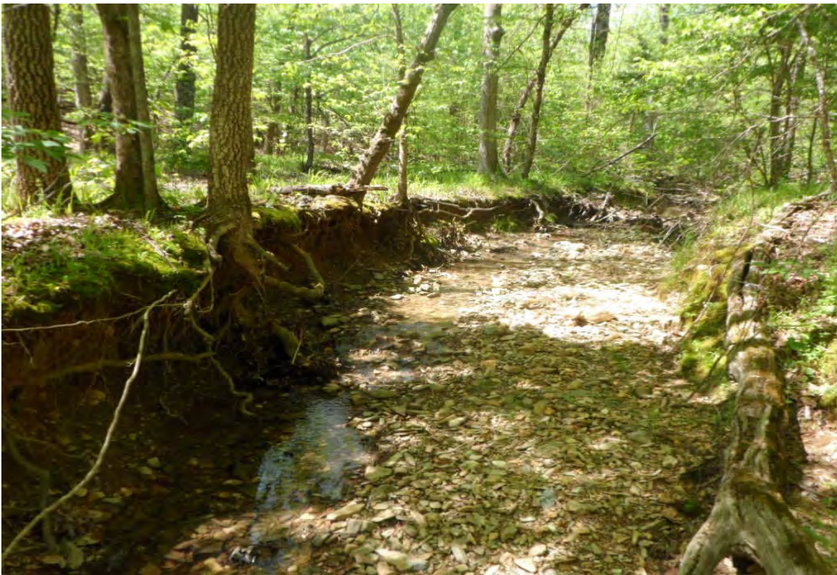
Section of unstable bank and proposed restoration location on Stream #3
